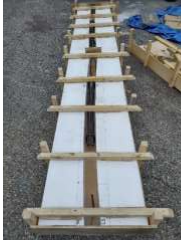
Fig. 4 Forms for curved UHPC beams
